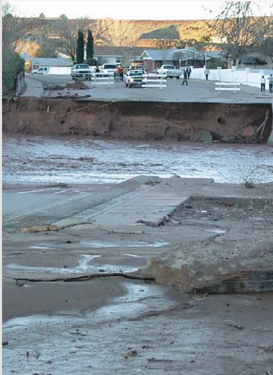
Valley View Drive Looking South
